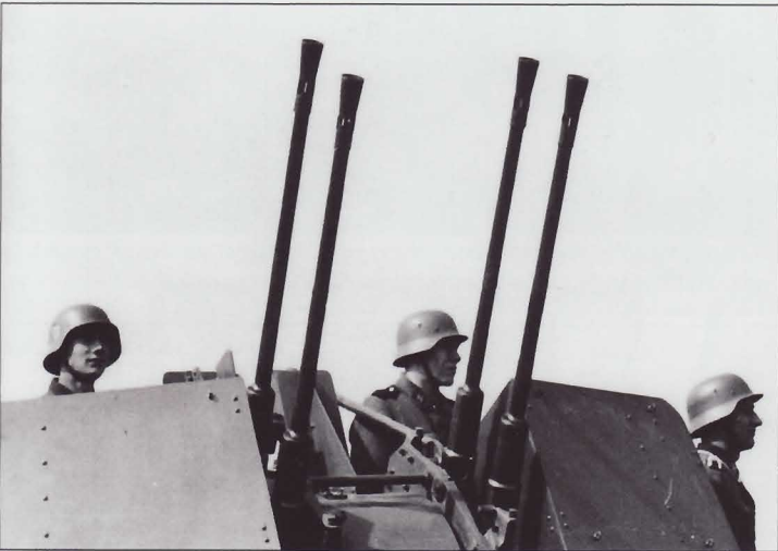
A four-barreled 2cm Flak38 anti-aircraft gun manned by an SS crew. This lethal weapon had a very impressive rate of fire of 1800 rounds per minute, and was effective against all kinds of targets up to 3000m away. It was a valuable weapon for frontline units protecting troop and vehicle concentrations against low-flying aircraft. The weapon was issued to Waffen-SS flak units in 1941, when the first flak battalions of the SS divisions were created, including those of "Das Reich", in May 1941.
