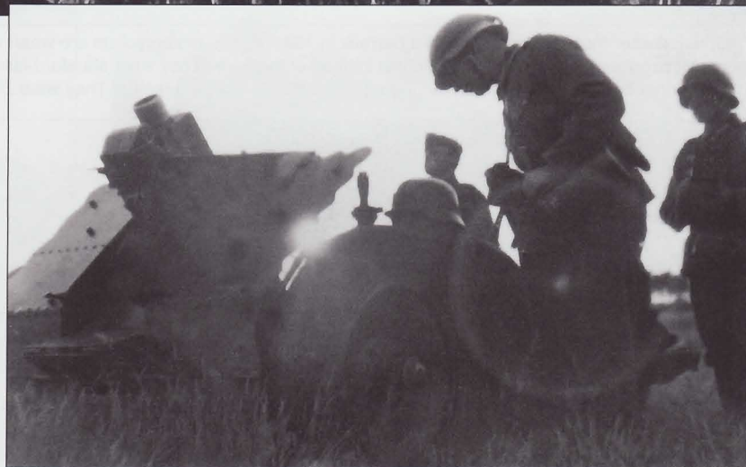
Prior to the invasion of Russia, an SS heavy weapons section is seen during a training exercise armed with a 7.5cm le.IG18 gun. In order to help conceal the weapon in open terrain, the gun's splinter shield has been camouflaged with foliage. The men exhibit an excellent display of infantrymen's combat equipment. A web battle pack carrier is attached to their Y-straps, as are the mess kit and shelter quarter. Note that all the infantrymen have the earlier type of camouflage straps around the M35 steel helmet. These were eliminated in 1940, but troops were still seen wearing them during the opening phase of Barbarossa.
