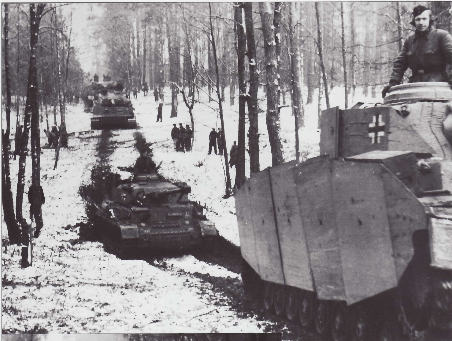
A column of Pz.Kpfw.IVs moving through a Ukrainian forest. The leading Pz.Kpfw.IV is a brand new vehicle complete with Zimmerit anti-magnetic mine paste and intact Schürzen. Note the vehicle following behind - the frontal plate of the tank's superstructure displays the "Das Reich" tactical sign.
