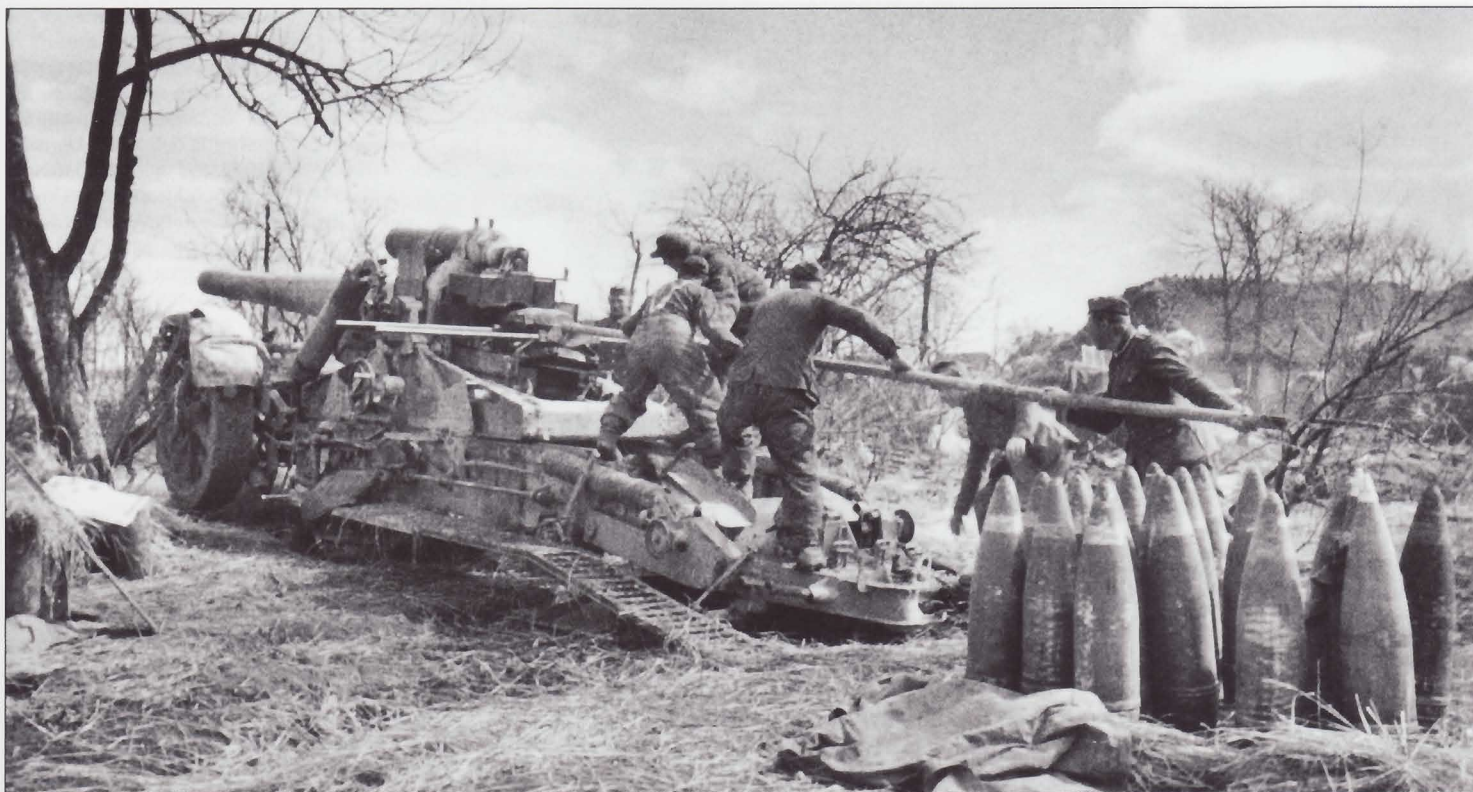
The strongest fire support in the Waffen-SS arsenal was the 21cm Mörser, seen here in early 1944. This photograph is a fine view of the gun and its projectiles. Note the size of the rammer needed to ram home the 150kg shell. These projectiles could be hurled some 20km into enemy lines with devastating
